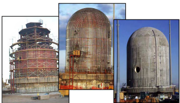
Figure 51 PCCY Model Construction
