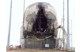
Figure 63 PCCY Model after the Structural Failure Mode Test
