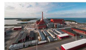
Olkiluoto EPR start-up delayed by final checks
