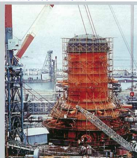
Primary Containment Vessel Under Construction (Unit No.1)
