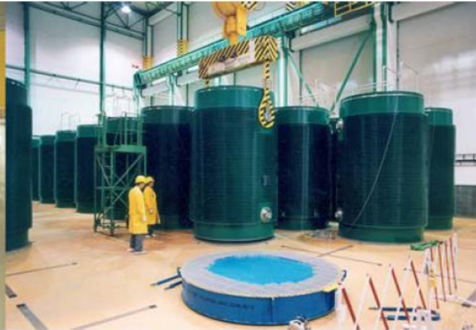
Dry storage facility at the Dukovany NPP (Czech Republic)
