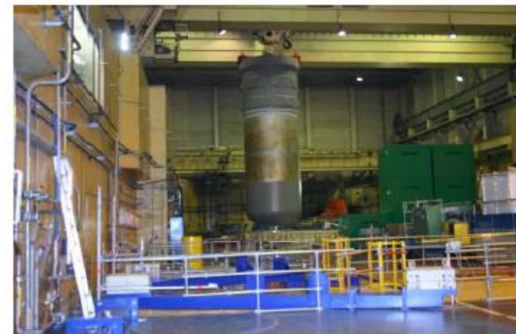
KGR reactor vessel removal and interim storage at Greifswald NPP
