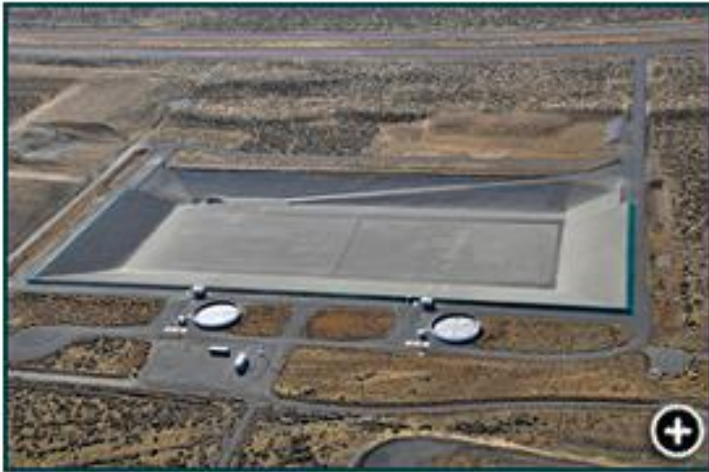
Figure 2. Integrated Disposal Facility.
